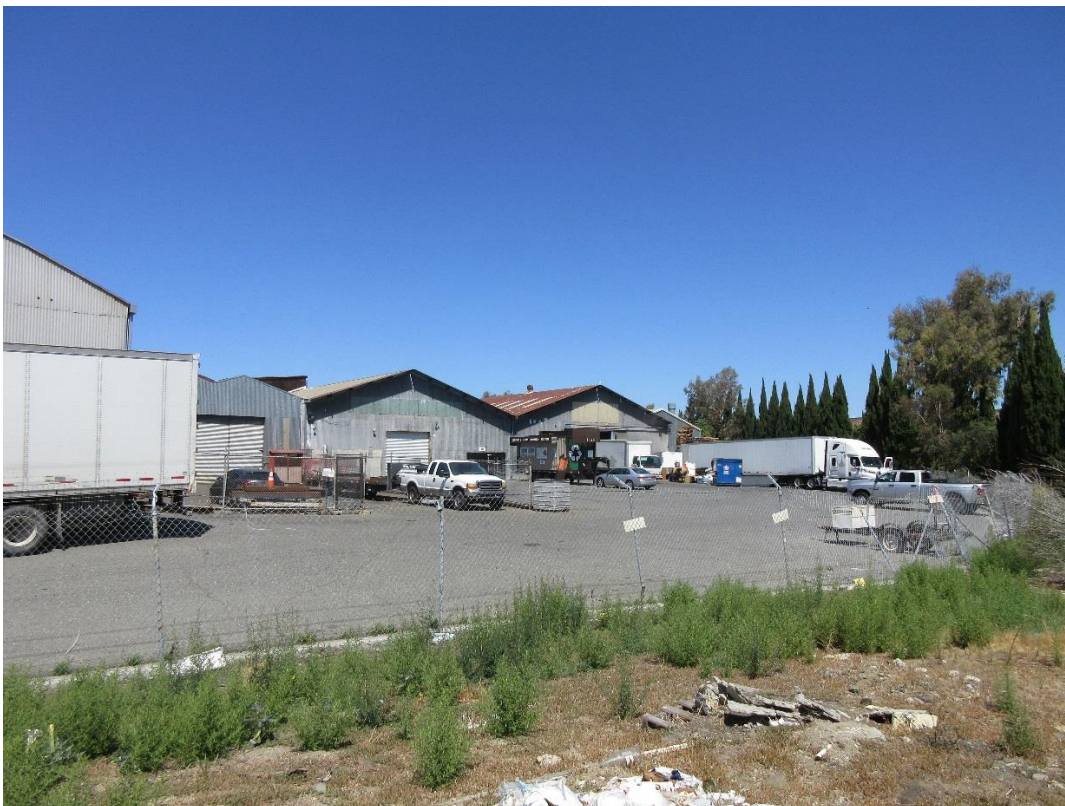
Photo 4.1-4: View of eastern side of project site, from the UPRR line, facing west.
