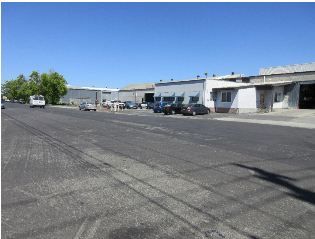
Photo 4.1-1: View of eastern portion of project site from Walsh Avenue, facing north.
