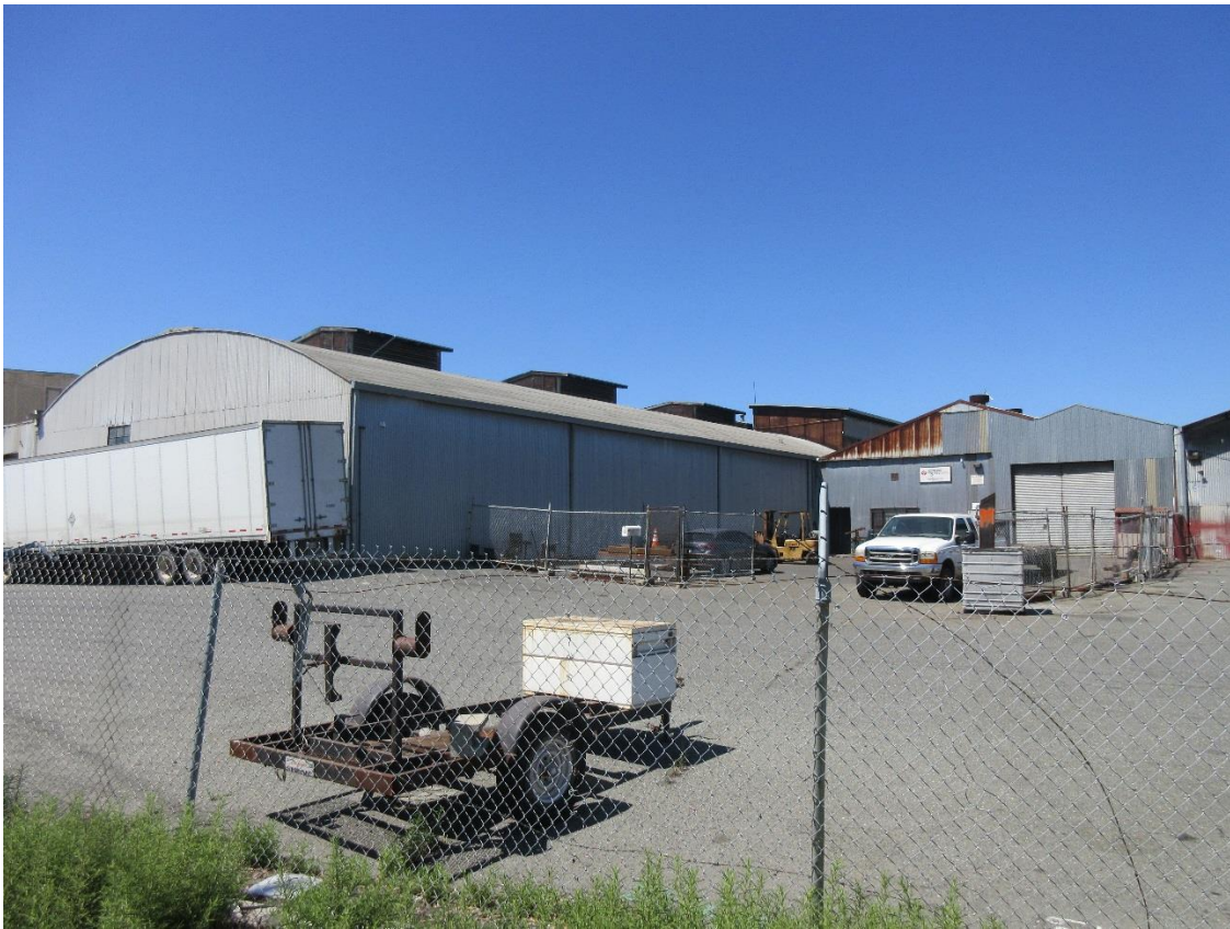
Photo 4.1-5: View of northern side of project site, facing south.
