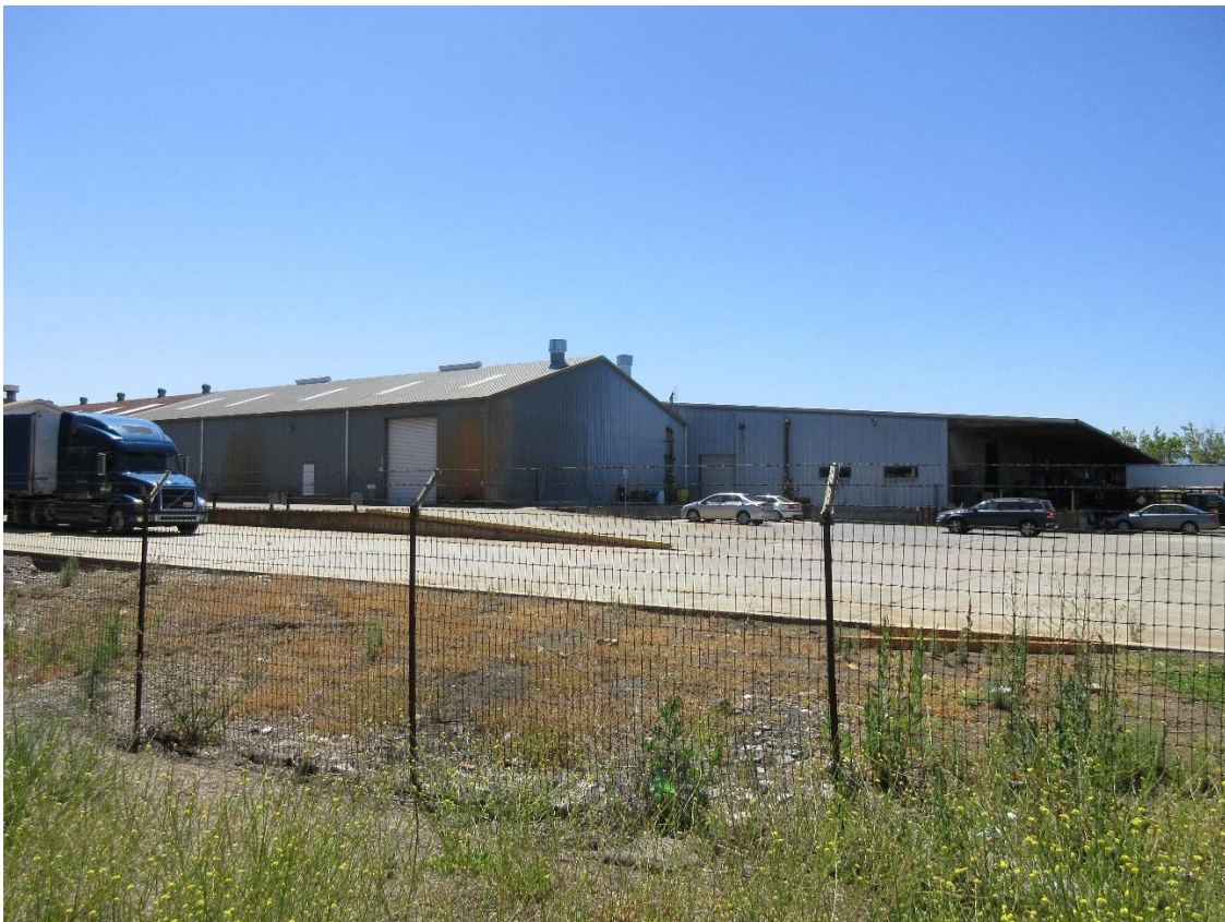
Photo 4.1-6: View of northern side of project site, facing southeast.
