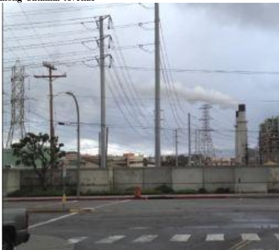
Figure 18: Another windy day (15 KTS). Same effect... exhaust plume blown down into neighborhood
