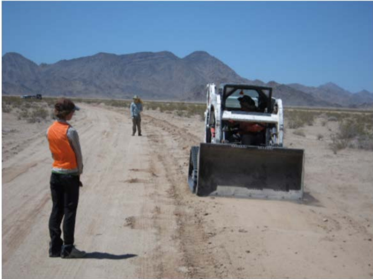
Figure 5 - Grade Restoration after Fence Removal
