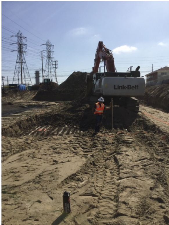
Excavation for 480V Auxiliary transformer depth ~EL61'
