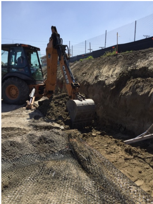
Backhoe excavating down to EL63 for conduit installation
