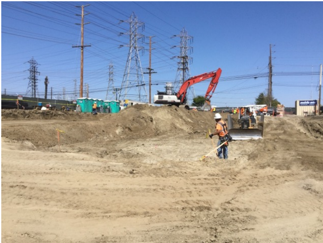
Excavator and dozer used for mass excavation
