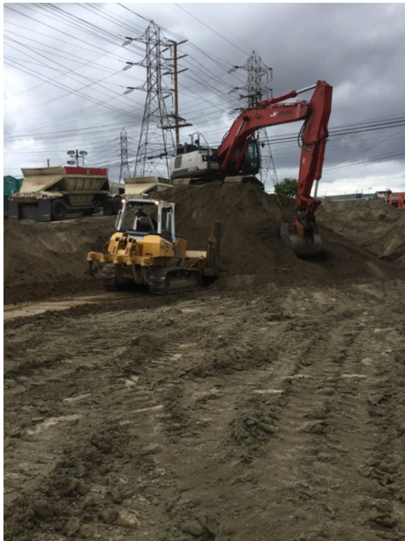
Excavator and dozer used for mass excavation
