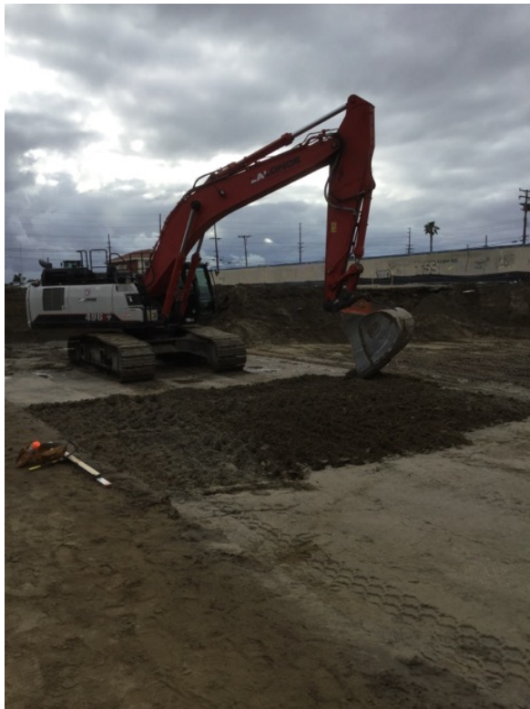
Excavator taking another foot off the grade to meet compaction.
