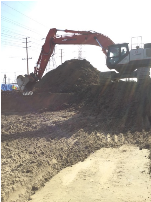
Excavator stockpiling sediment from cut, ~8bgs
