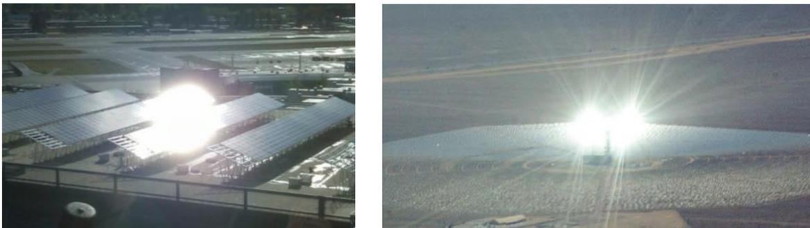
**Figure 1. Examples of solar glare. Left: PV system at Manchester-Boston Regional Airport viewed from the air-traffic control tower. Right: Glare from Ivanpah CSP plant viewed from an aircraft.**
