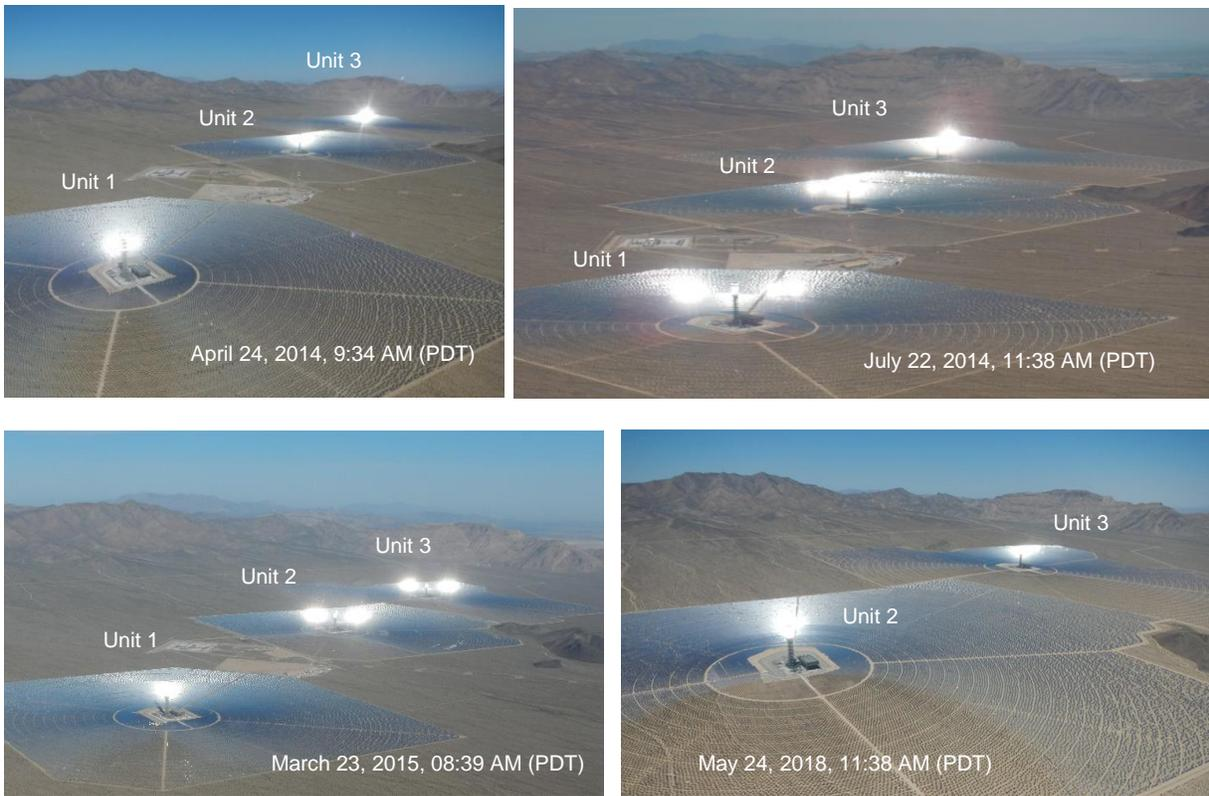
**Figure 32. Sequence of photos of glare at Ivanpah taken on different dates looking northwest. Note that on May 24, 2018, Unit 1 was not operational.**
