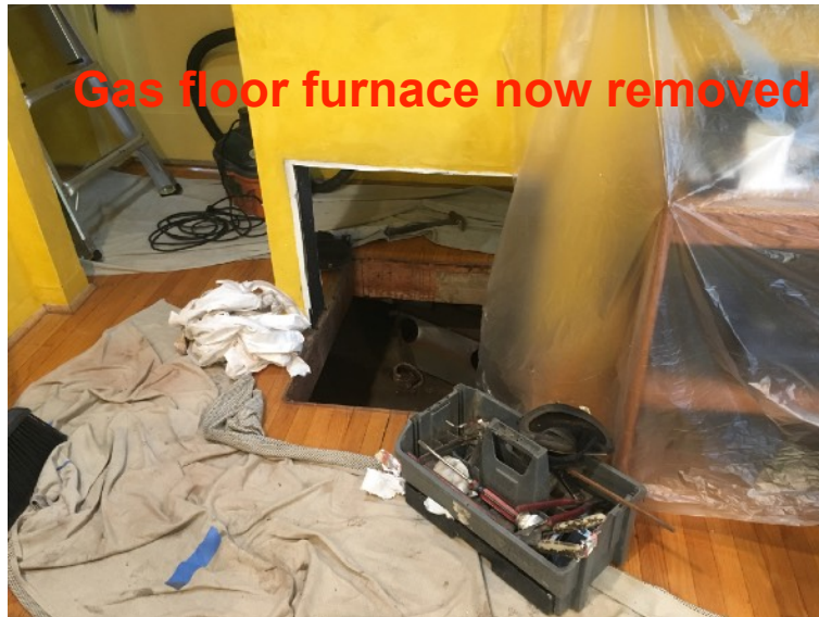
1948 gas floor furnace in living room
