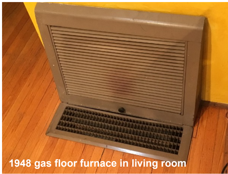
Gas floor furnace now removed
