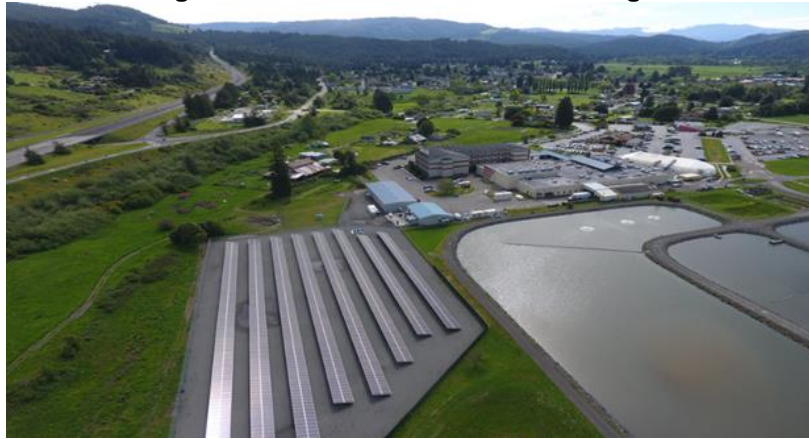
Figure 43: Blue Lake Rancheria Microgrid
