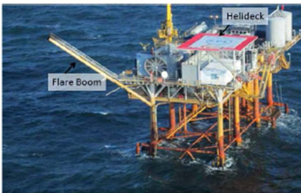
Figure. SS208H showing the helideck and flare boom.
