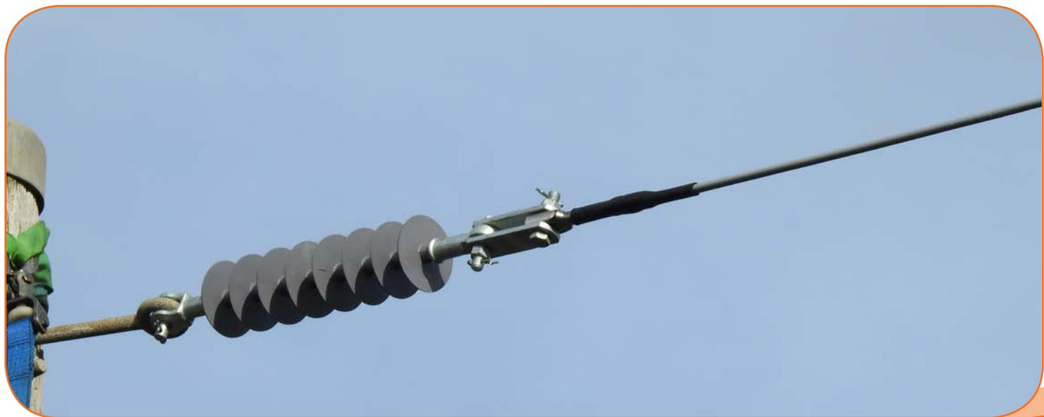
Figure 6: Installed ACS covered conductor on SWER asset
