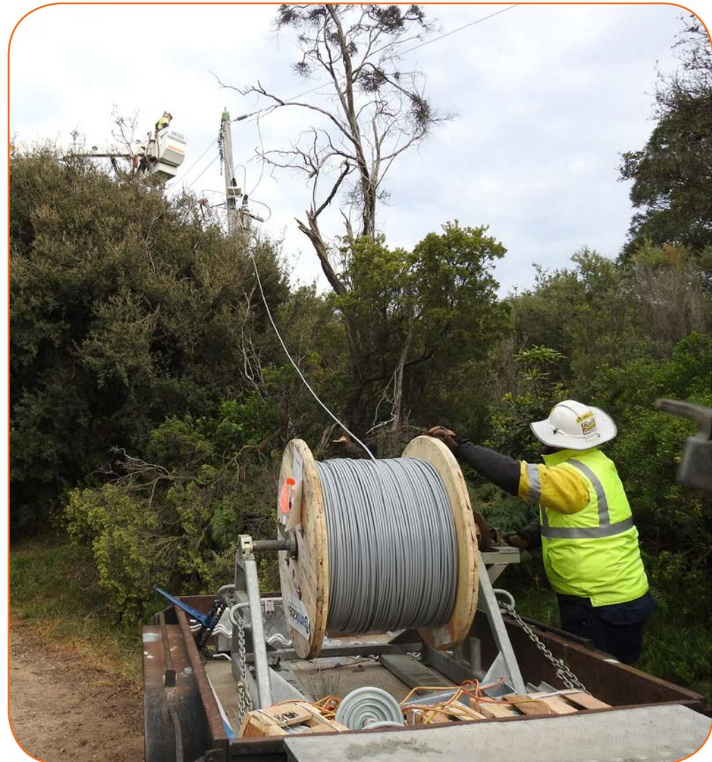
Figure 5: Stringing ACS covered conductor on SWER
