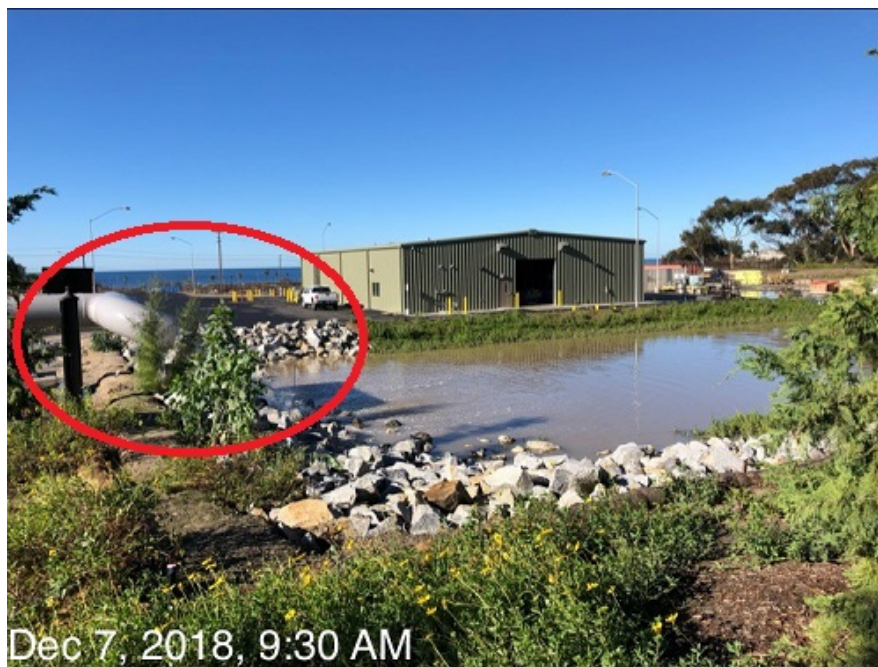
Photo 6. Stormwater from the Construction Site and Pump Station is being sent to the bioswale. Photo taken 12/7/18, facing west.
