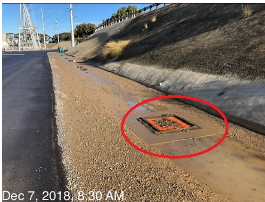
Photo 4. Drain covers have installed in preparation for rain events to prevent debris from entering the stormwater system. Photo taken 12/7/18, facing north.
