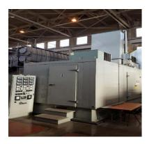
Vernon owns and operates two natural gas-fired combustion turbine units (H. Gonzales Generating Station #1 and #2), which are also located within the City of Vernon. The H. Gonzales natural gas-fueled combustion turbines are Allison 571-KA combustion turbines, rated at 5.75 MW each. The combustion turbine units began commercial operation in 1988. Each of the units is restricted by air quality regulators to run on natural gas for no more than six hours per day.
