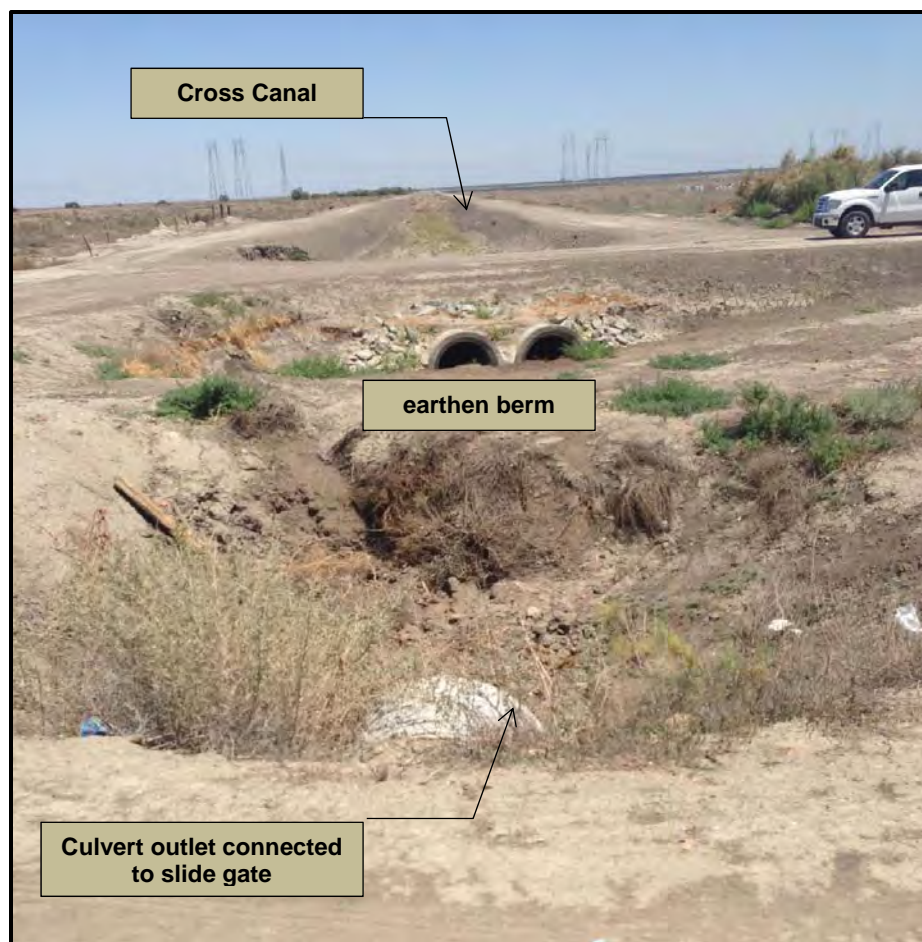
Photo 2. Looking east from the Kern River Flood Control Channel slide gate culvert. Note the earthen berm that separates the culvert outlet and the West Side Canal (located on the far-side of the earthen dam). The two culverts in the center of the picture connect the West Side Canal to the Cross Canal.
