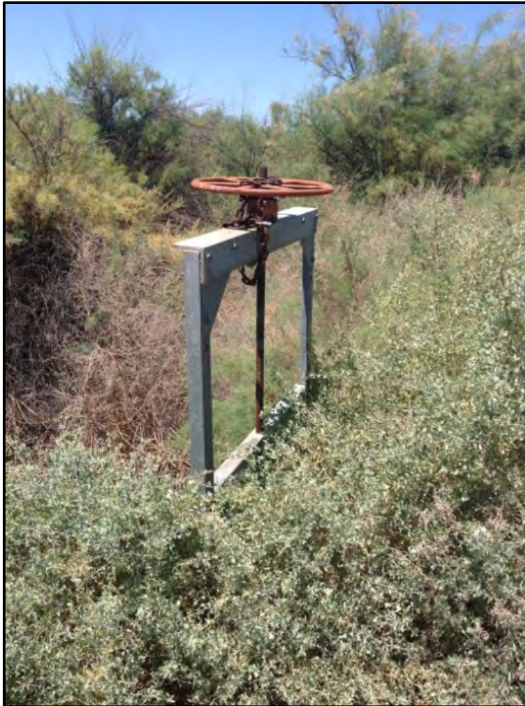
Photo 3. Looking north at the slide gate that controls diversion of water from the Kern River Flood Control Channel to the West Side Canal/Cross Canal location shown in Photo 2.
