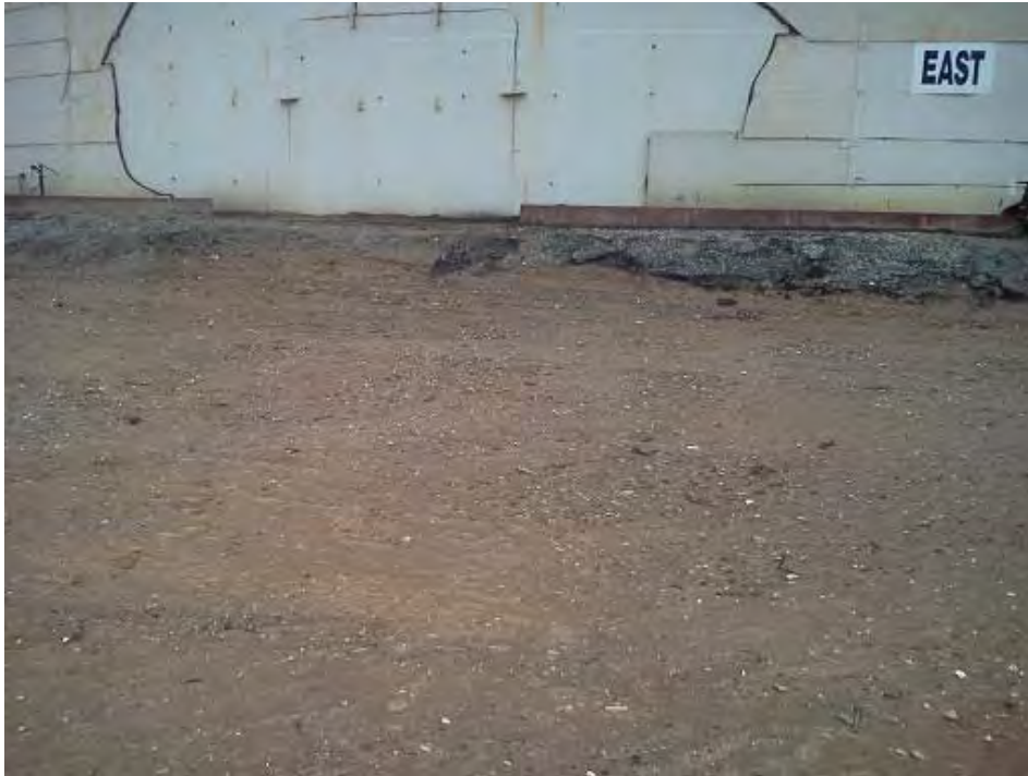
Photo 1: Location of soil pit prior to excavation.
