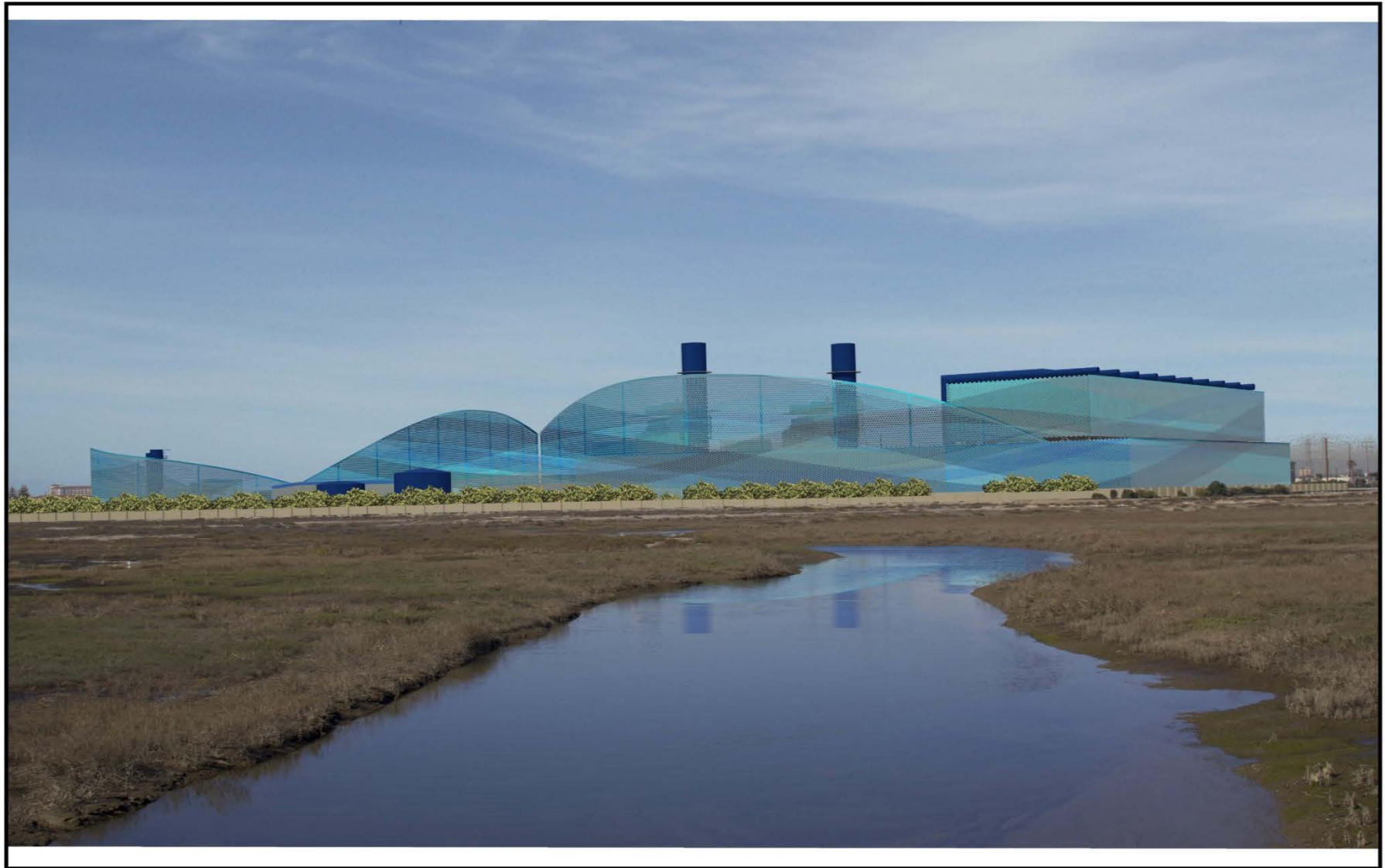
CALIFORNIA ENERGY COMMISSION - SITING, TRANSMISSION AND ENVIRONMENTAL PROTECTION DIVISION SOURCE: TN #210763
