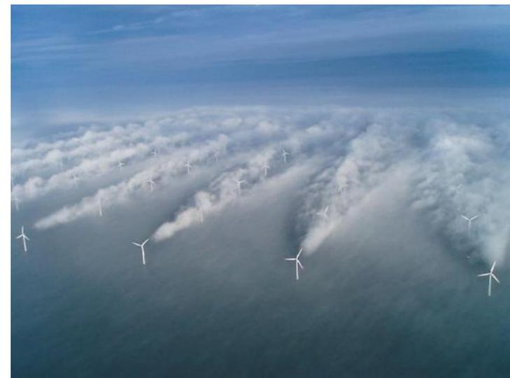
Wake Interaction at Horns Rev Offshore Wind Farm
