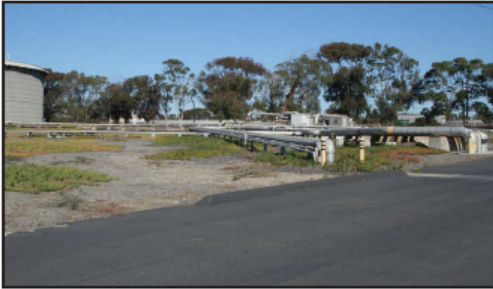
KOP 10- Existing View from Encina Power Plant Site
