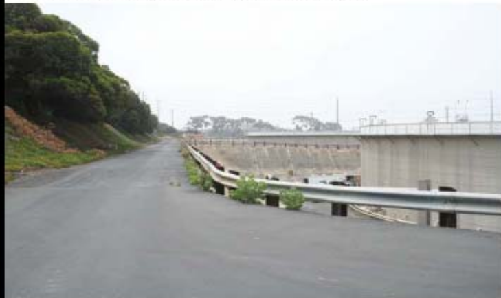
2. Internal road on project site looking southeast
