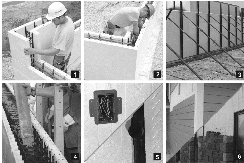
Figure 2: ICF Construction Process
