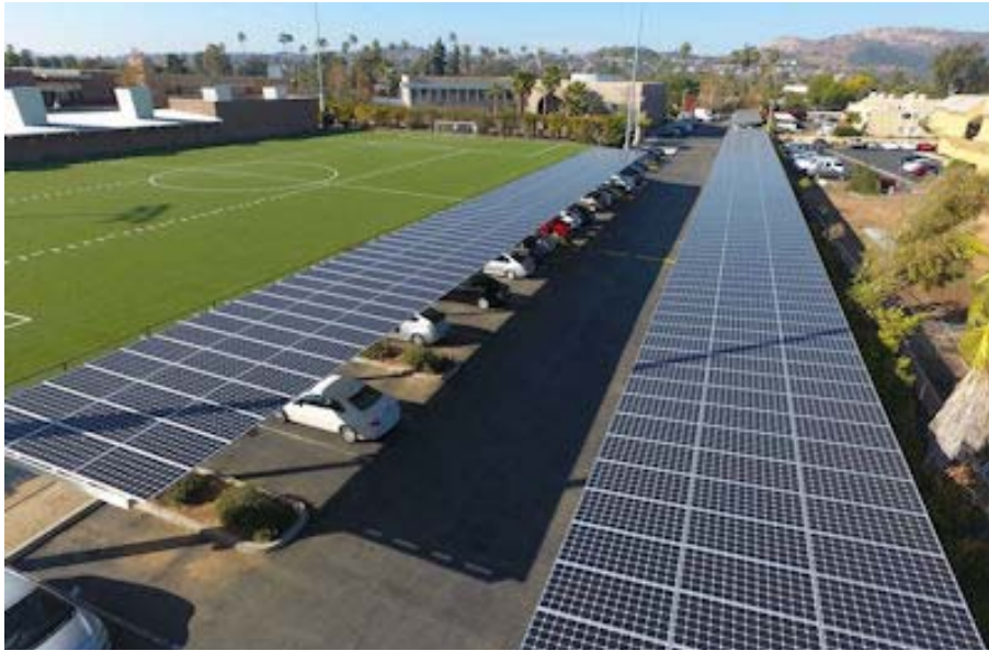
Photo 11: The Solar for Schools Program Will Install Carport Shade Structures
