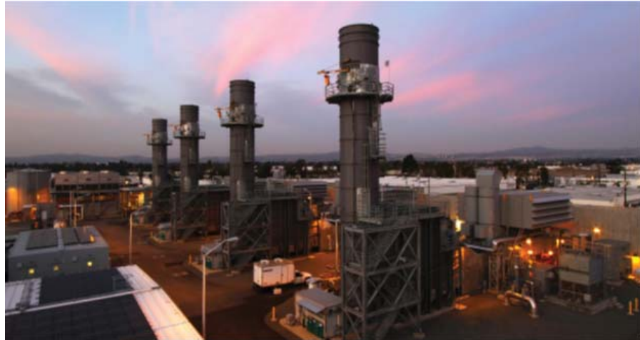
Photo 3: Canyon Power Plant
