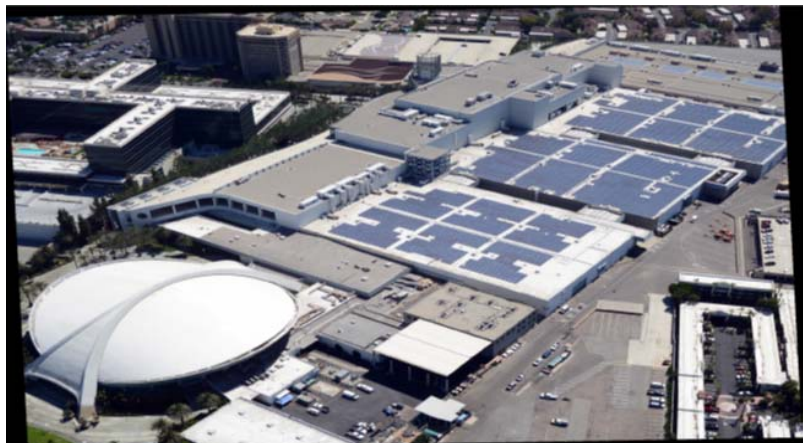
Photo 5: The 2.4 MW Anaheim Solar Energy Plant at Convention Center
