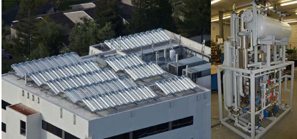
a. Solar thermal and absorption chiller to provide hot water and cooling at a hotel
