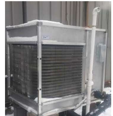
f. Gas-fired heat pumps for water and air conditioning in restaurants
