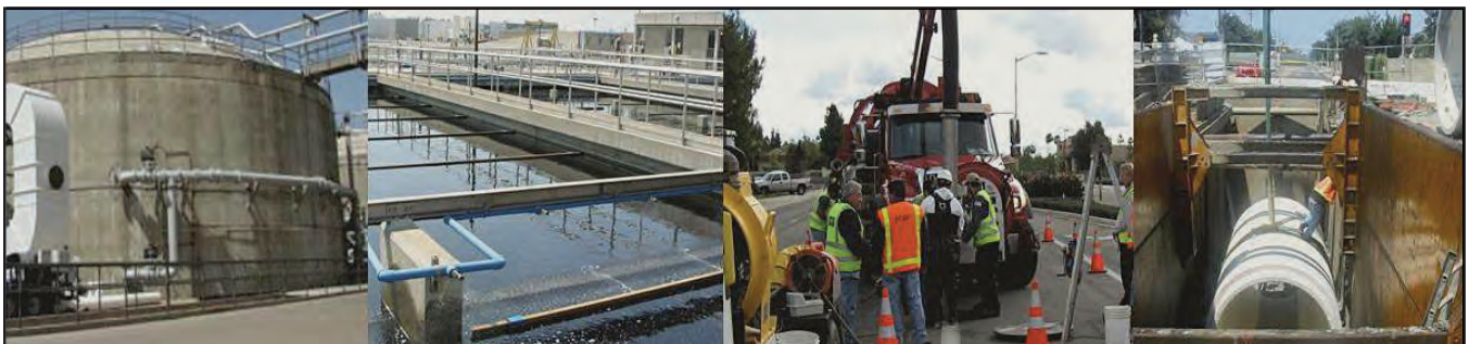
OCSD owns and operates $6.2 billion in infrastructure assets. Through these assets OCSD collects, treats, and either reuses or safely discharges 210 million gallons per day of wastewater.
