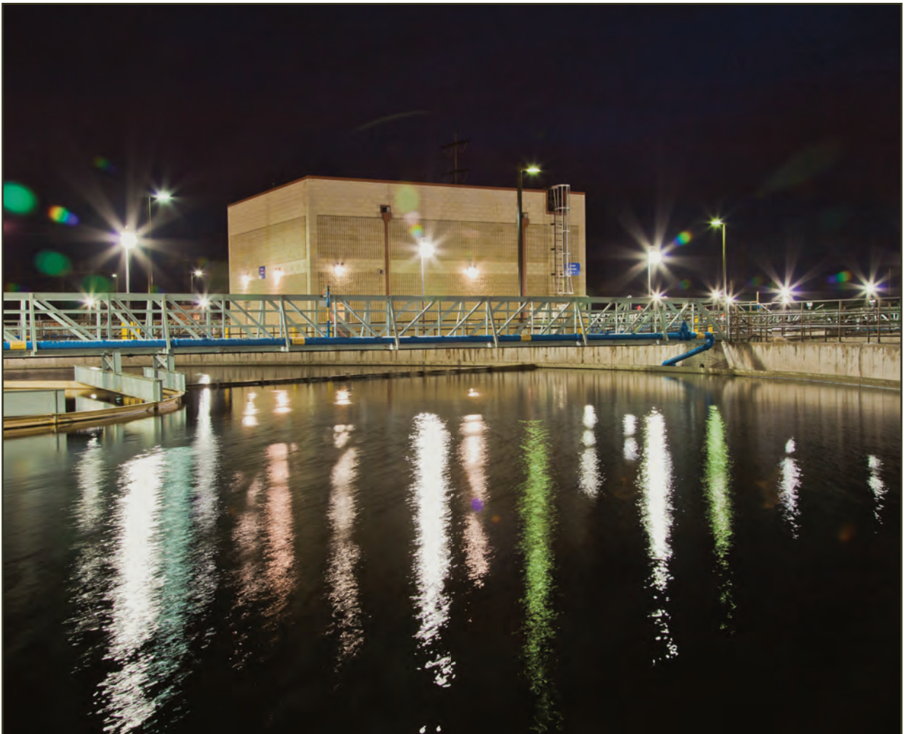
The activated sludge secondary treatment facility was the final project to meet the EPA Secondary Treatment Consent Decree. This facility increased secondary treatment capacity at Plant No.1 by 60 million gallons per day.
