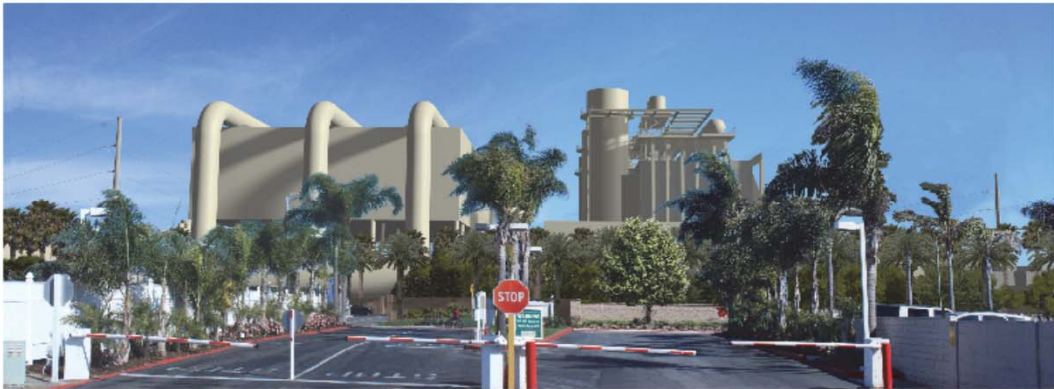
B. Simulated view depicting appearance five years after completion of project development
