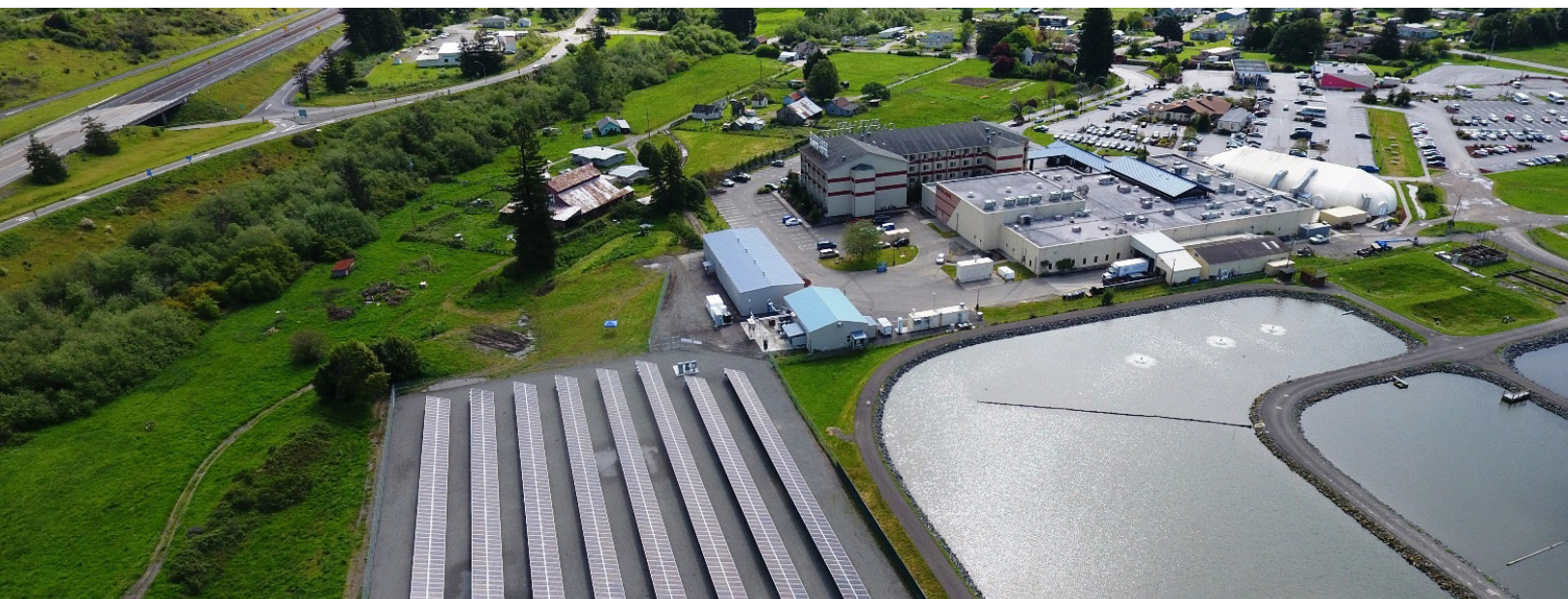
In 2017, the The Blue Lake Rancheria completed an award-winning microgrid project that includes a 420-kilowatt solar array and nearly 1 megawatt-hour of energy storage. The system can automatically disconnect from the grid when needed to continue powering critical infrastructure, preparing the local community for the impacts of wildfires, earthquakes, and tsunamis.
