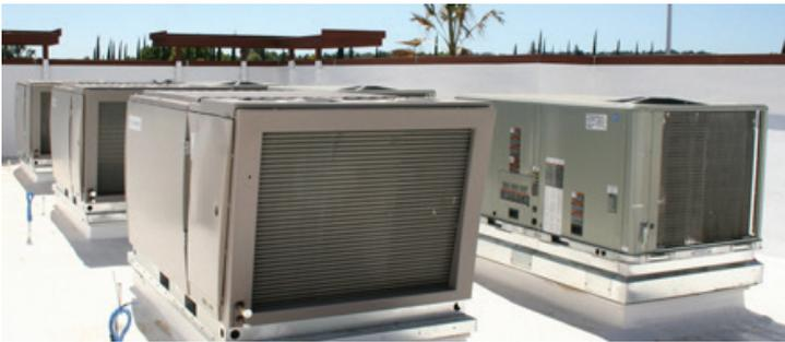
Figure 10 shows the Ice Bear storage commercial air conditioning unit. These devices actually provide both peak and energy savings, because they “make cold” at night, when temperatures are lower and the chilling units operate more efficiently, offsetting the usual “round-trip losses” associated with electrical energy storage.
