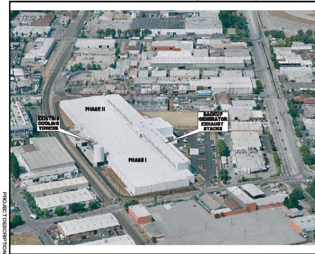
CALIFORNIA ENERGY COMMISSION - SITING, TRANSMISSION AND ENVIRONMENTAL PROTECTION DIVISION SOURCE: SPPE November 2011, Fig. 2-6
