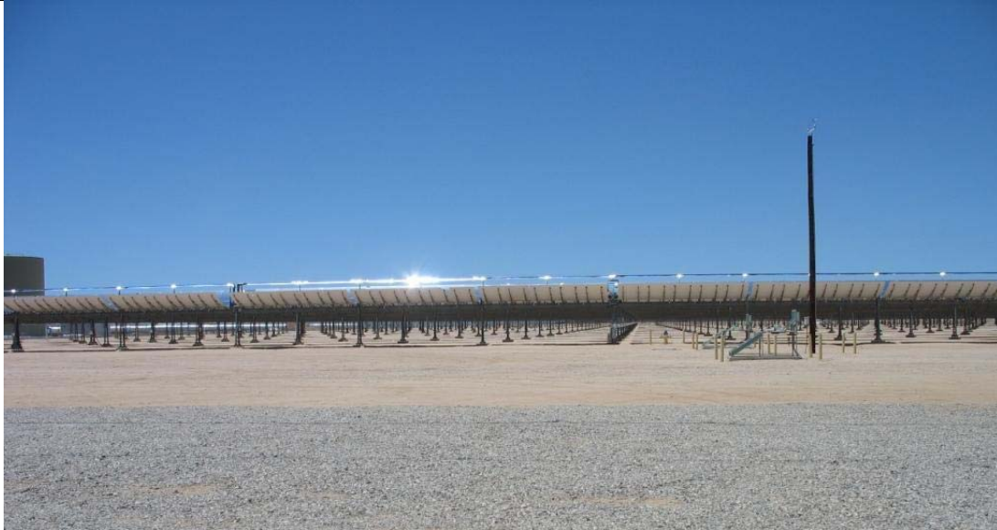
Figure 2. Ground Level View of Direct Reflection from the 70 mm Glass Heat Collection Element (HCE) at the Focus of the Parabolic Mirror at the SEGS Power Plant. There will be a wind fence surrounding the facility that will prevent most such reflections from being visible from a ground level observer.
