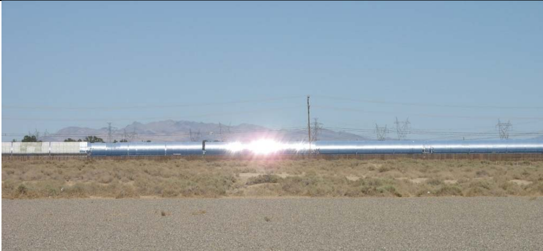
Figure 3. Ground Level View of Reflection and Scattering from the HCE Tube at the SEGS Power Plant. Note the Diffuse Glow due to Scattering Along the Entire Length of the HCE Tube. There will be a wind fence surrounding the facility that will prevent most such reflections from being visible from a ground level observer.
