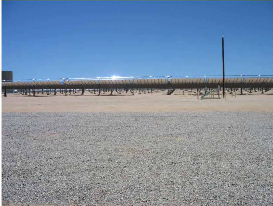
In this photograph, the mirrors are pointed vertically. The most intense reflection is from a joint connector on the normal to the observer. Reflections off the individual joints in the HCE tube are visible. Note the limited extent of glow and lack of reflection from the operating HCE tube visible on either side of the normal.
