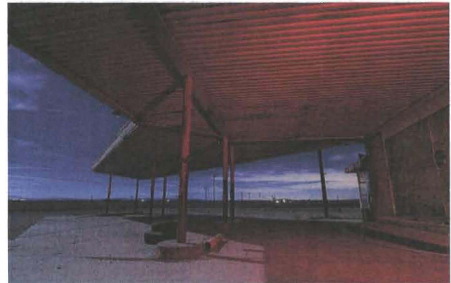
Lockhart General Store and Gas Station 1951, Canopy as it remains today 2010
