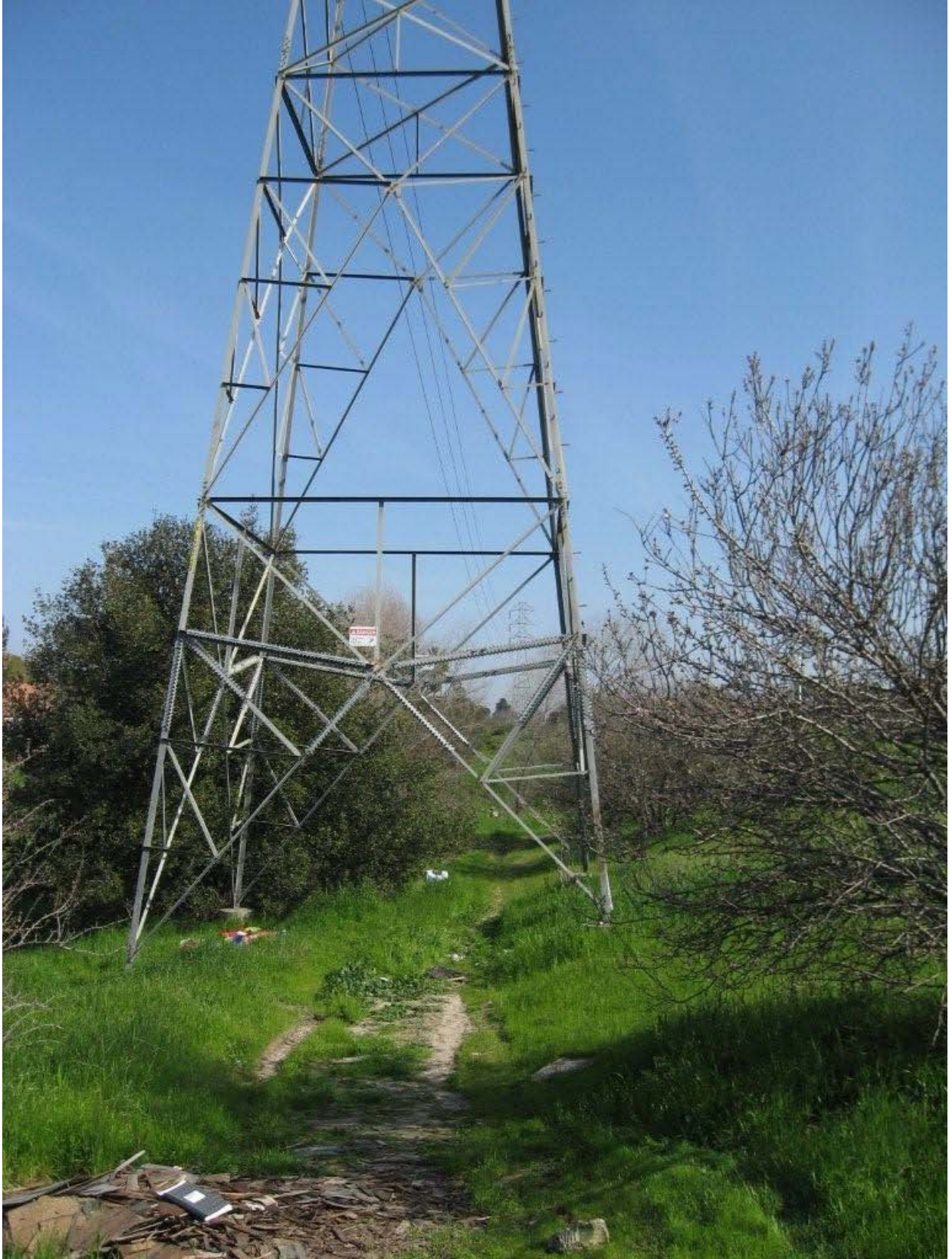
Tower #16 with interior live oak to be removed, 2/17/10.
