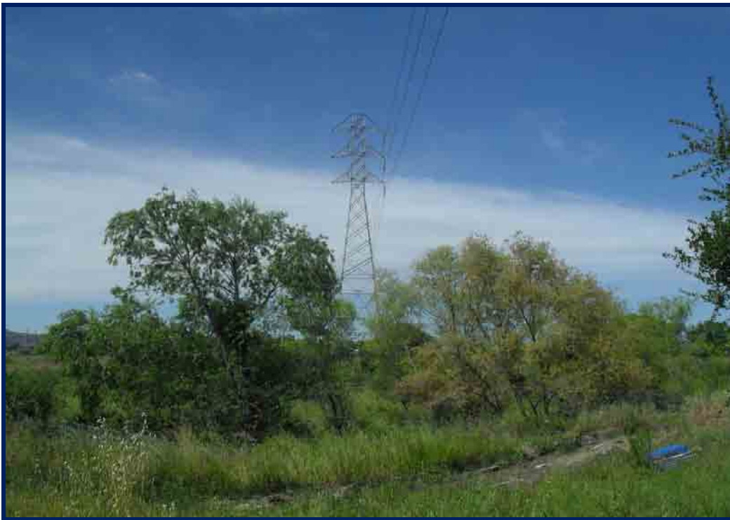
FIGURE 4 Looking west at existing 60-kV transmission lines lattice tower along unnamed creek west of housing development. Red willow riparian habitat.
