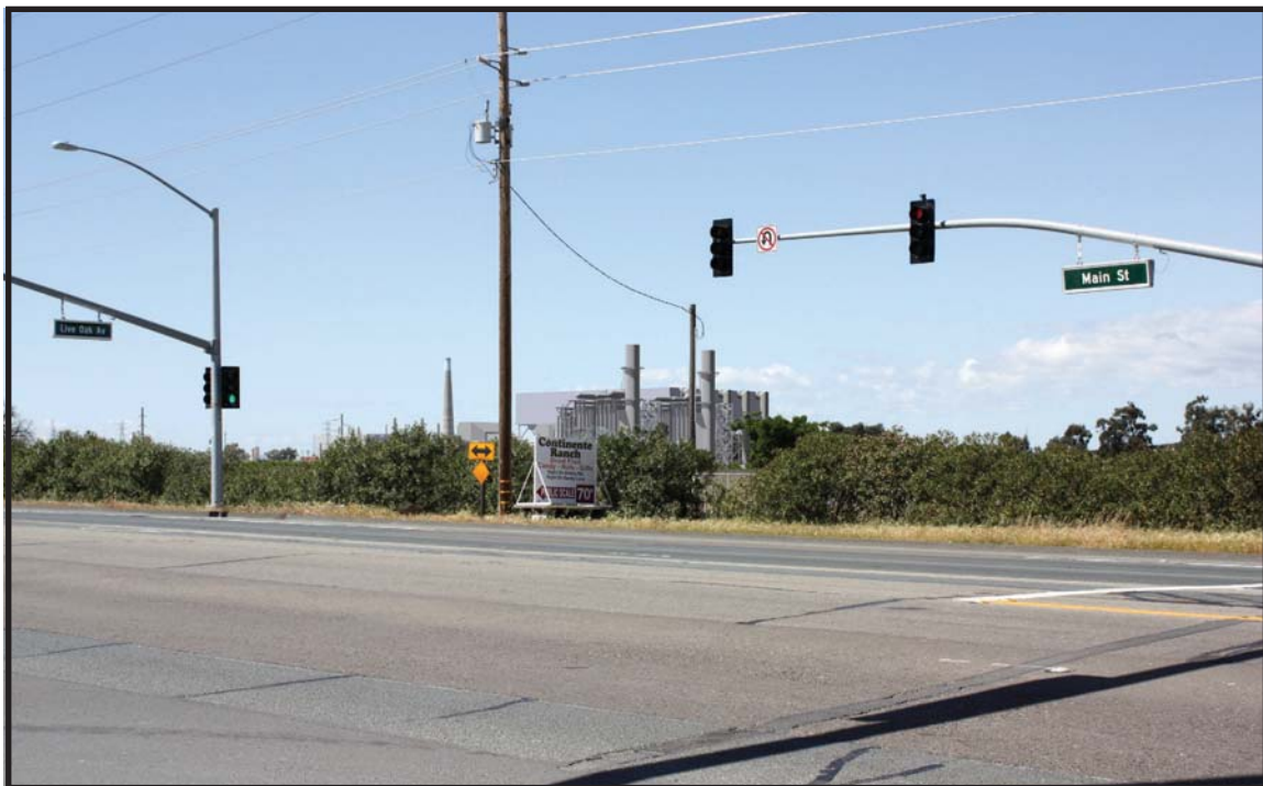
4b. View from KOP-3 with simulated project and landscaping five years after installation.
