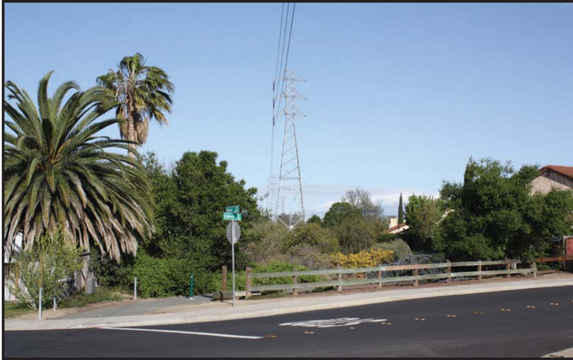
8a. View to the east from intersection of Viera Avenue and Oakley Road, in Antioch (KOP-7). This segment of the transmission corridor includes a pedestrian path, the entrance to which is visible in the center of this view.
