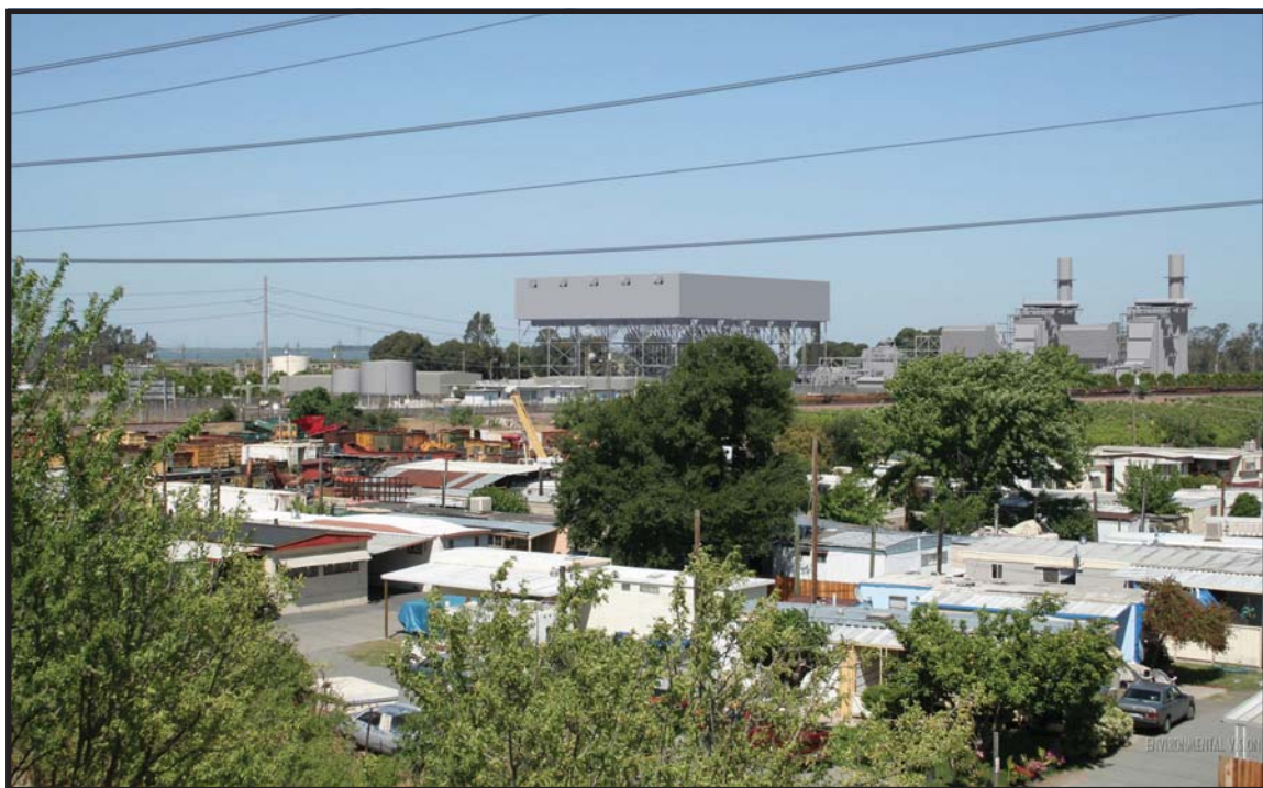
3b. View from KOP-2 with simulated project and landscaping five years after installation.
