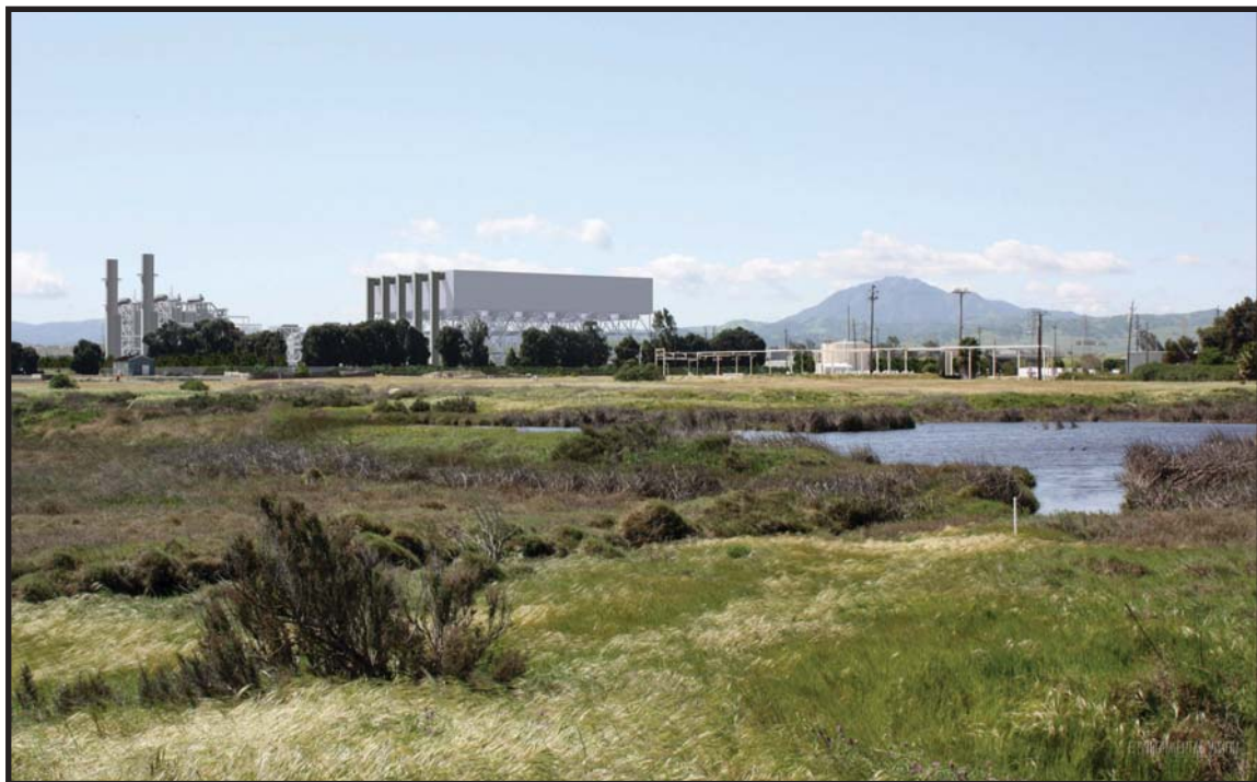
6b. View from KOP-5 with simulated project and landscaping five years after installation.
