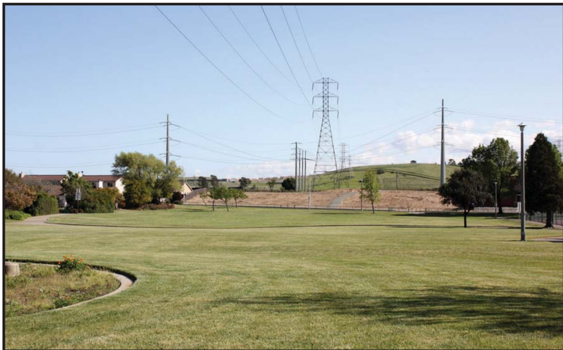
7b. View from KOP-6 with transmission corridor replacement simulated.
