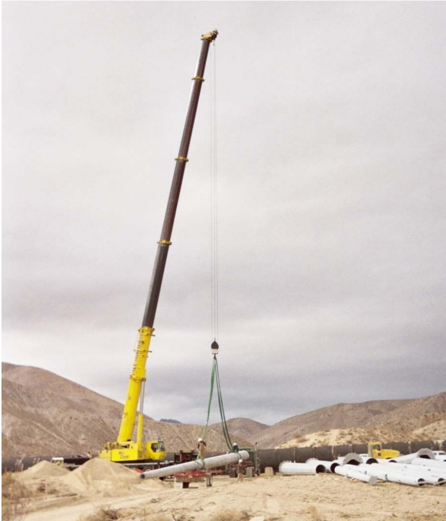
Figure 4. Concrete pole being lifted off delivery truck/trailer
