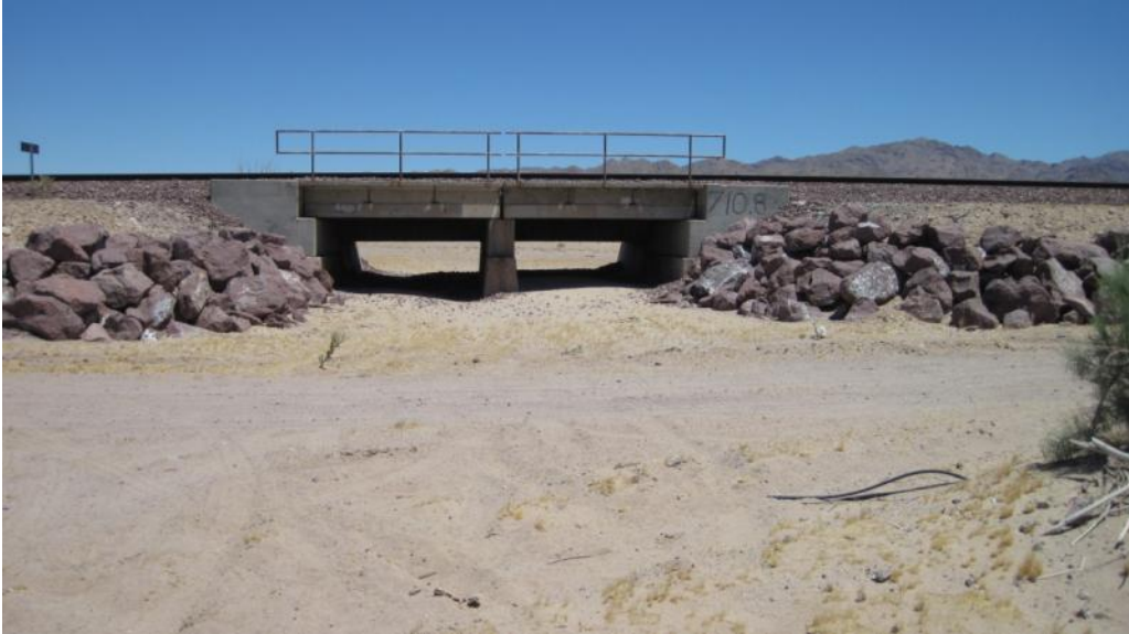
Trestle 3 - Photo taken looking upstream
