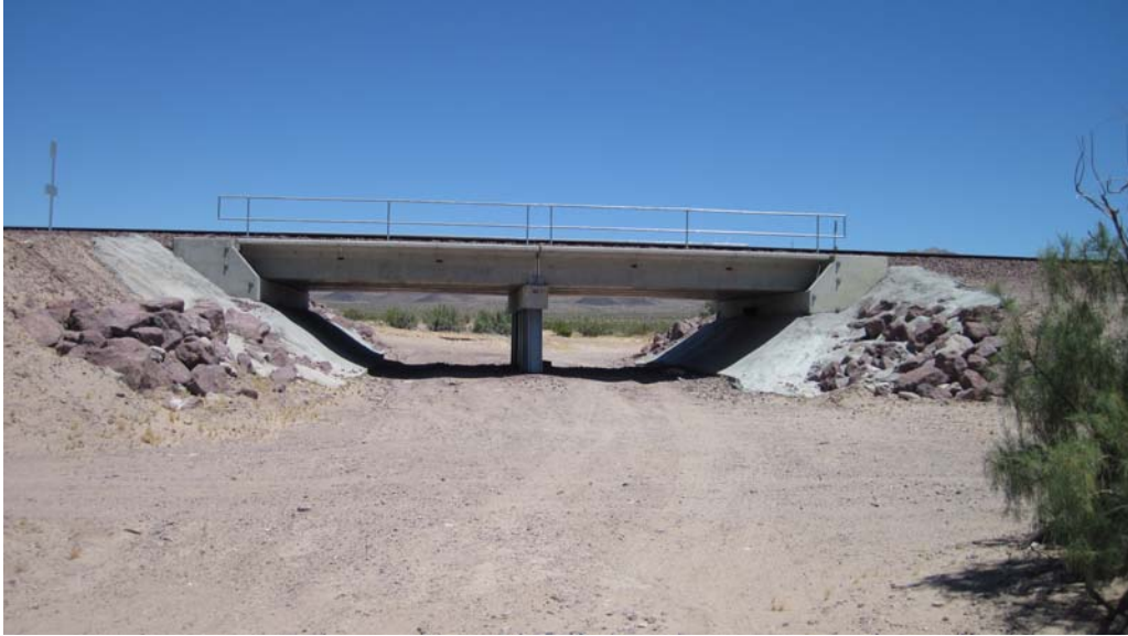
Trestle 4 – Photo taken looking upstream
