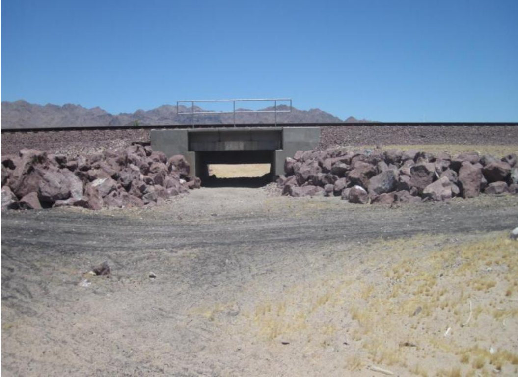
Trestle 7 – Photo taken looking upstream
