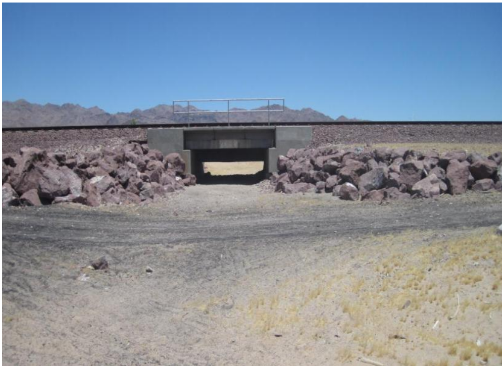
Figure 3.5b. Looking upstream through Trestle 7.
