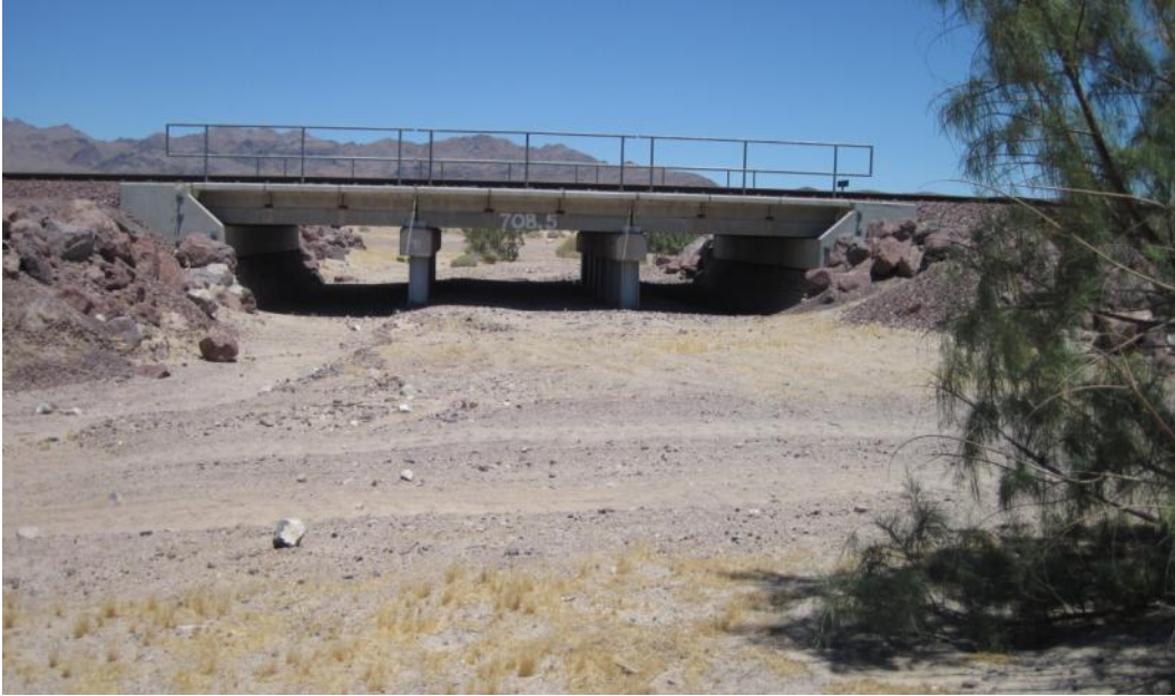
Trestle 8 – Photo taken looking upstream
