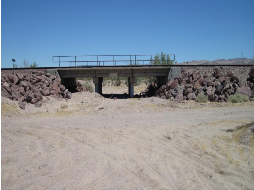
Trestle 2 - Photo taken looking upstream
