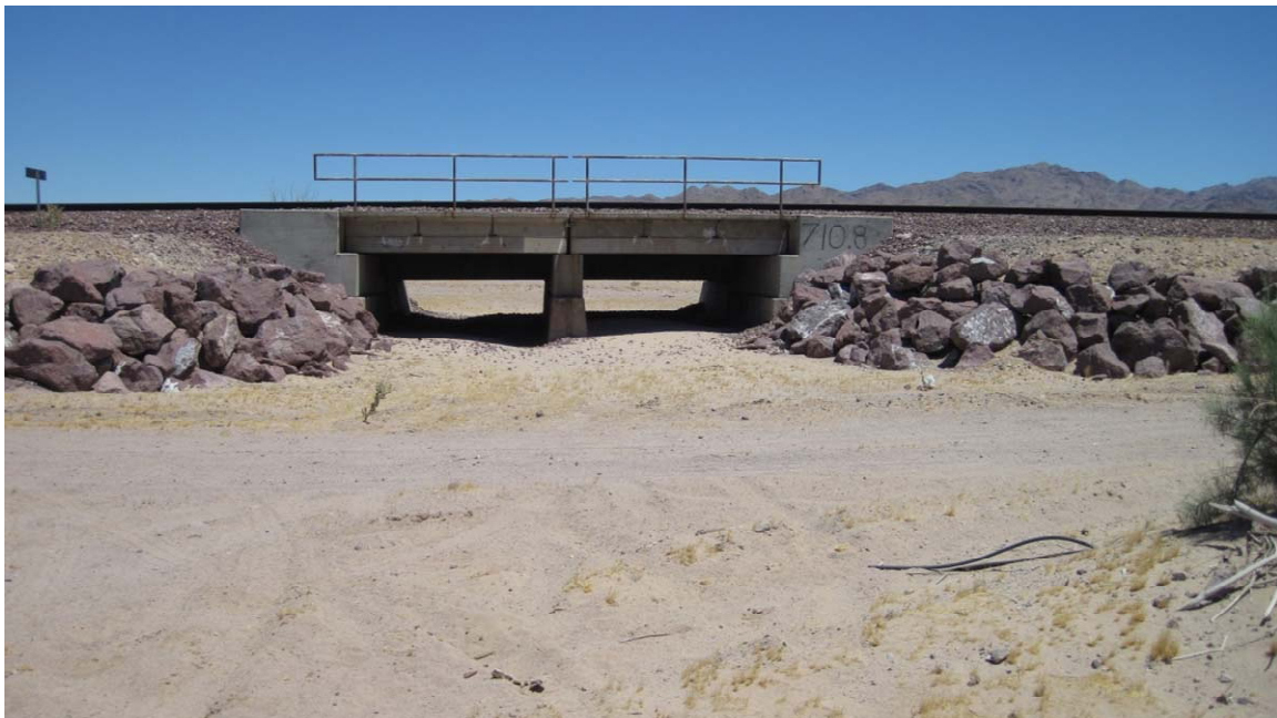
Figure 3.4b. Trestle 3, looking upstream (north).
