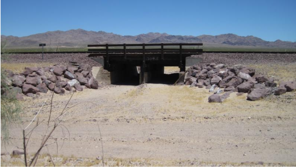
Trestle 5 – Photo taken looking upstream
