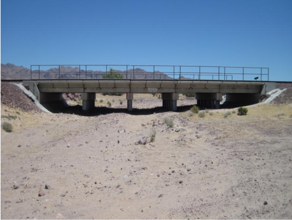
Trestle 6 – Photo taken looking upstream
