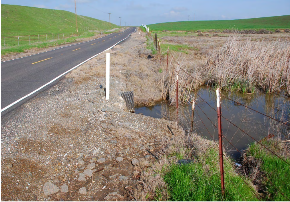
#5. Water line alignment at Drainage 4 (D-4), looking north. Pipeline will be installed under the D-4 culvert using pipe ramming.
