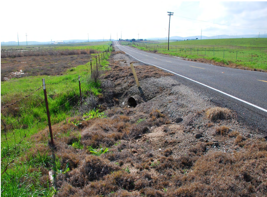
#5. Water line alignment at Drainage 4 (D-4), looking north. Pipeline will be installed under the D-4 culvert using pipe ramming.
