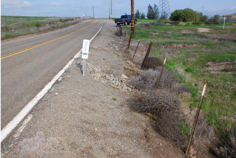
#3. Water line alignment near Drainage 2 (D-2), looking north. The pipeline will be buried just right (east) of the culvert (indicated by the white marker) within the right-of-way.
