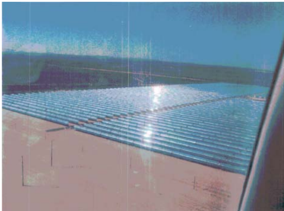
Figure Two: Image of a parabolic trough plant from a low flying airplane 1
