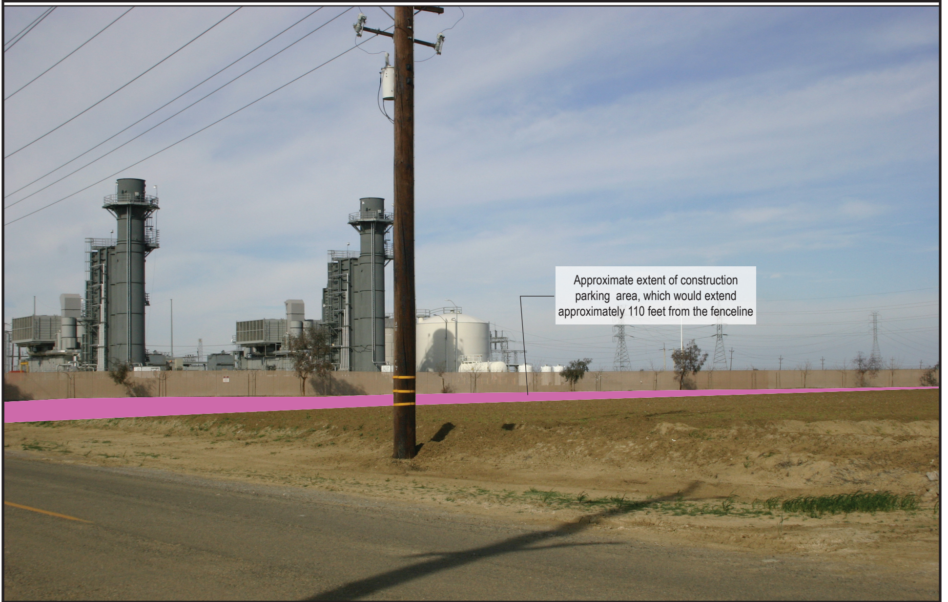
A. View to the northeast of the project site from 25th Avenue. This location is not a Key Observation Point. The area to be temporarily disturbed by construction parking would occupy the entire area in front of the HPP in this view, extending approximately 110 feet from the existing fence line. The distance between the fence line and the wooden pole visible in the immediate foreground (center view), is approximately 300 feet. Beyond the HPP, but in front of the lattice transmission towers visible in the center-right portion of this view, is the location of the proposed construction laydown area. Construction equipment and activities at that location could be visible from this viewpoint. Both the parking and laydown areas will be temporarily disturbed; upon completion of construction, all equipment and materials will be removed from the temporary parking and laydown areas.
