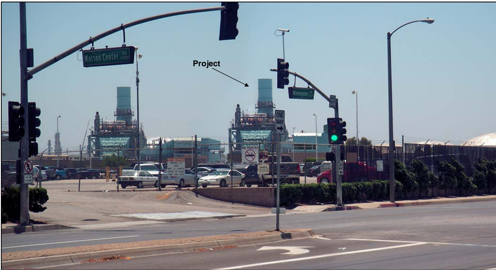
Watson Cogeneration Steam and Electric Reliability Project - KOP 1: Simulated View of BP Watson from KOP 1
