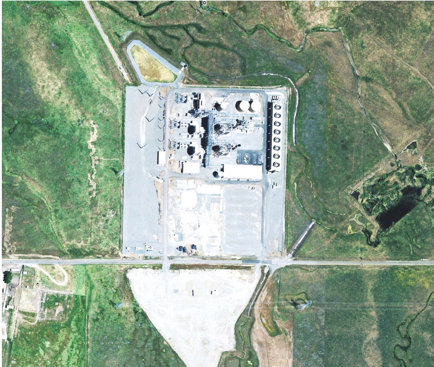
Figure 1-2. Site Aerial View
