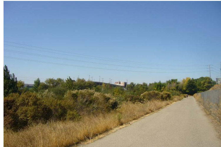
8. View of the central portion of the reconductoring project area from the eastern bank of the Guadalupe River, looking north. The lines span across the river channel.
