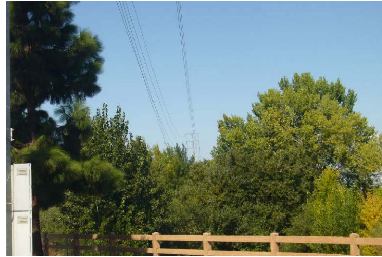
6. View of the central portion of the reconductoring project, looking northeast along the Guadalupe River. The lines here span across the Guadalupe River and its riparian canopy.
