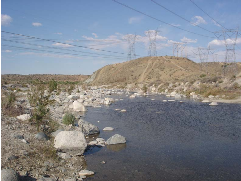
Photograph 1. Little Rock Creek survey area, April 21, 2009: looking north. Wooden H-Frames are proposed location of Transmission Line Segment 2.
