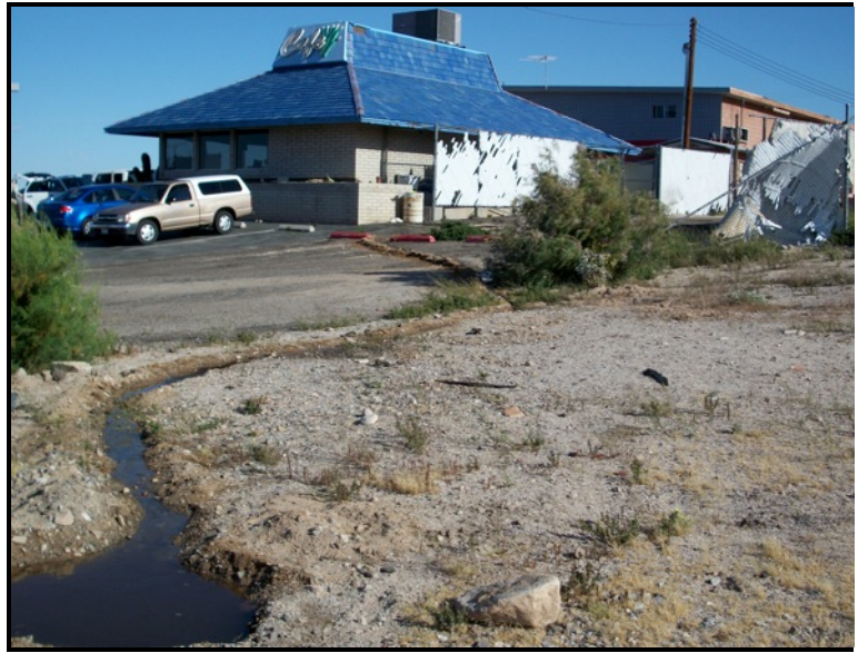
Photo 2: Sewage stream. The foreground building is a closed restaurant. The building in the back is the Texaco station.
