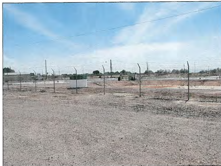
Photo C: View of treatment ponds from parking lot on Project site.
