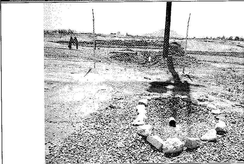
Photograph 9 - Recently installed stormwater drainage in the parking lot.
