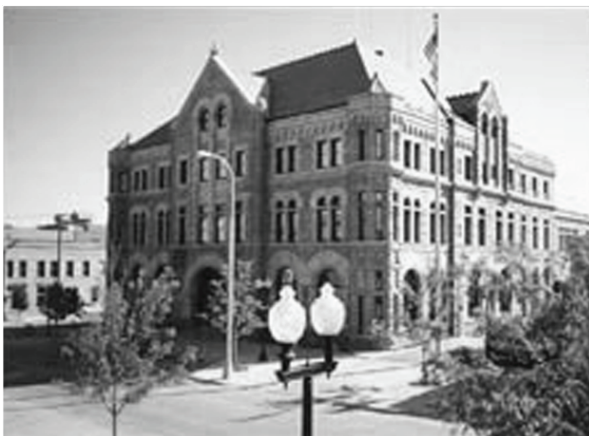
US District Courthouse, Sioux Falls, SD
