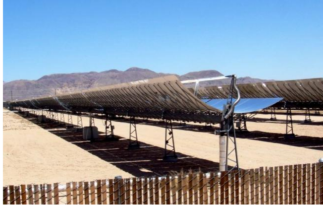
Parabolic trough technology as used in Daggett, CA (Sunray Energy, Inc.)
