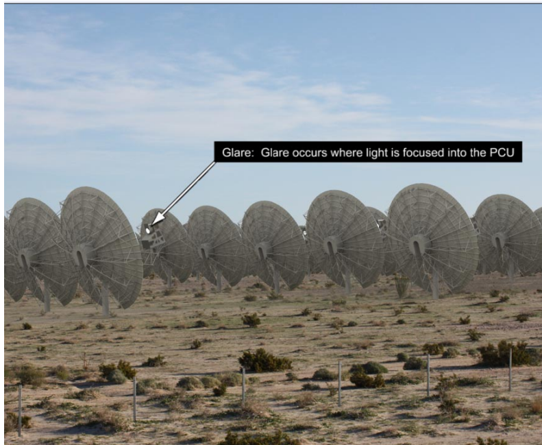
Figure 2 Schematic showing primary source of glare on SunCatcher™ system
