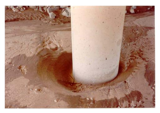
Figure 1. Local scour around bridge pier
