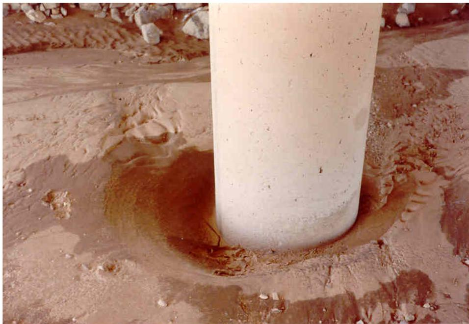
Fig. 33. Local scour around a bridge pier
