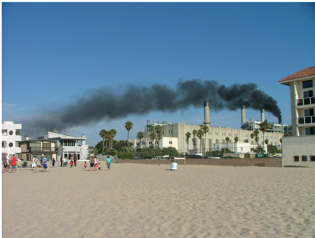
Photo 3: AES plant upset condition shows emissions blowing down into residential area
