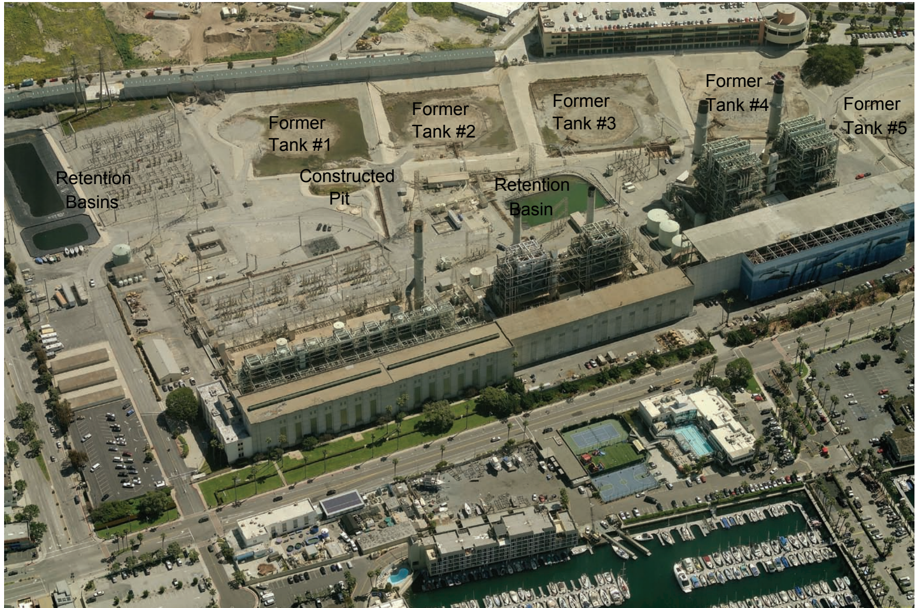
FIGURE 1 Photograph of Existing Site AES Redondo Beach Energy Project
