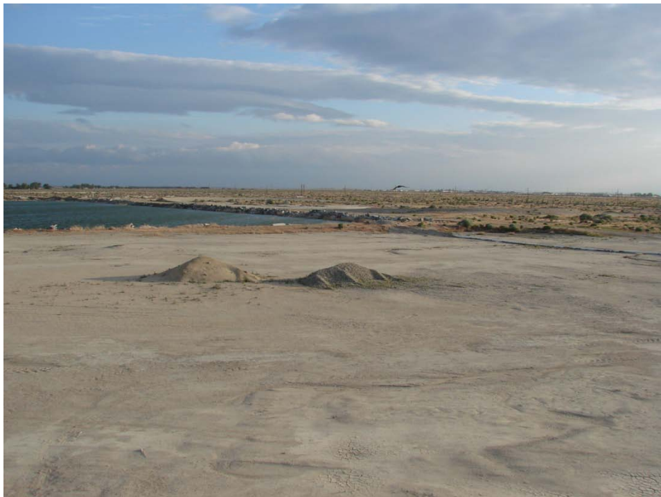
Northeast Corner Looking South - 5/17/10
