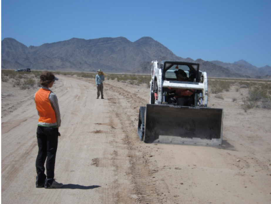
Photograph 7 - The “Bobcat” was used to restore grades to existing conditions with cultural and biological monitoring.
