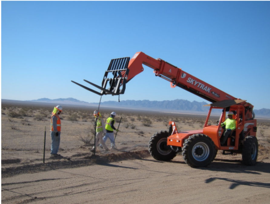
Photograph 1 – Typical fence removal process with extended-reach forklift
