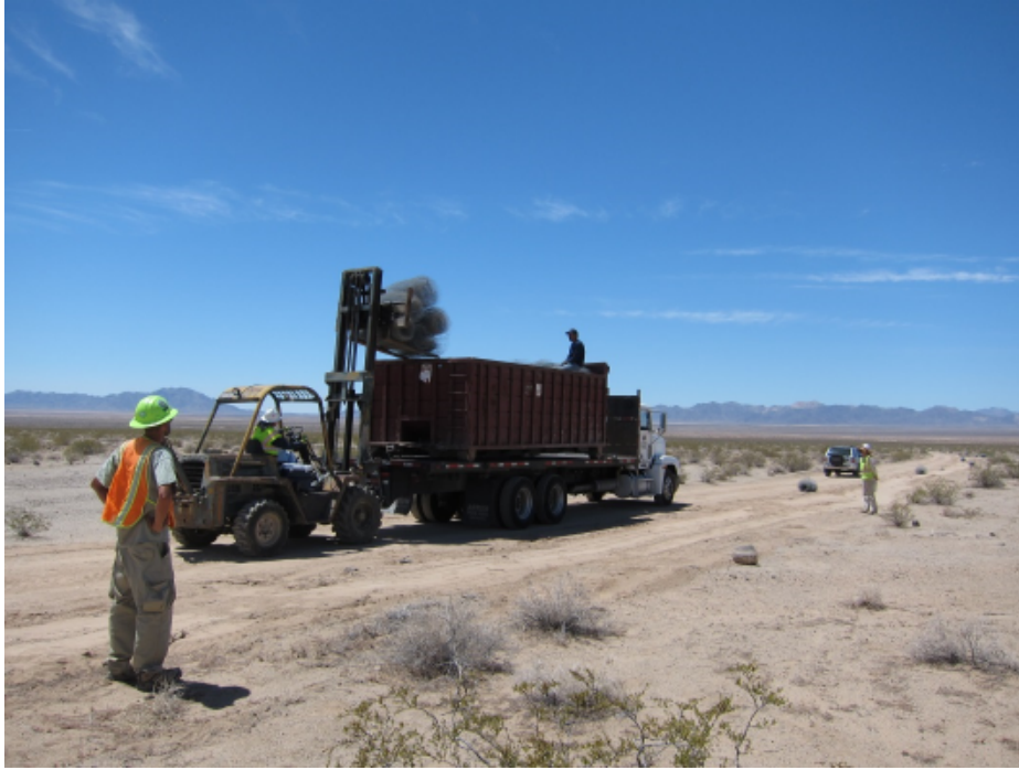
Photograph 9 – The desert tortoise fence being loaded onto a tractor and removed from site.
