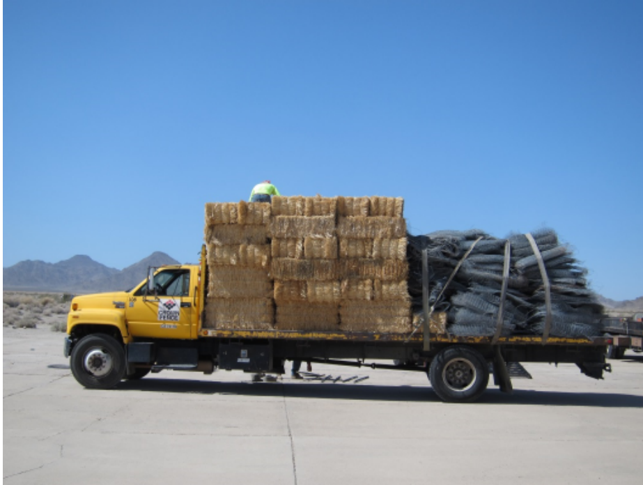
Photograph 11 – Removal of the Stormwater BMP's and desert tortoise fence from site
