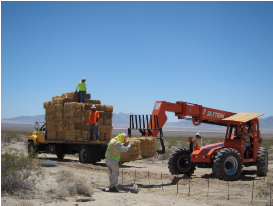
Photograph 10 – Removal of the Stormwater BMP's from the site
